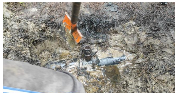
L-R: Two you young men scooping out sand and water and Valve fully revealed
