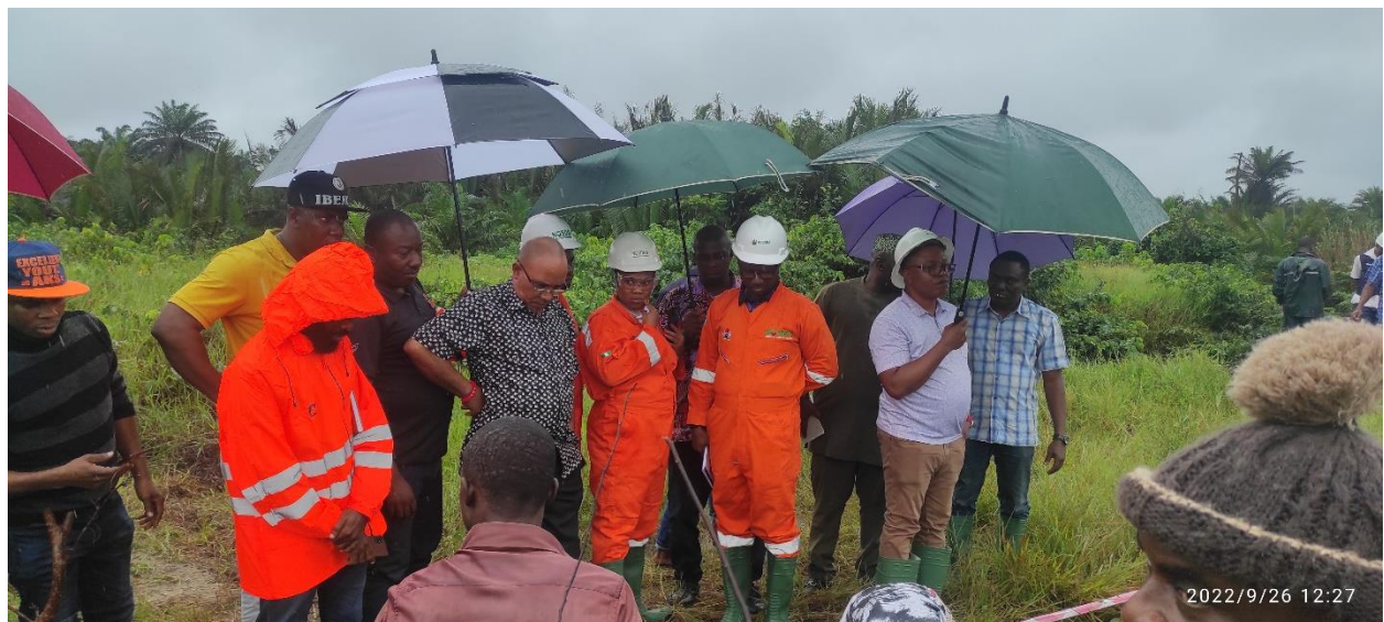
The JIT observes and ask questions to UERL as two young men scoop out sand and water to reveal the full extent of the pipeline and valve
